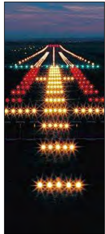
Figure 2-3 - Typical CAT II Runway Lighting
